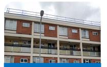
Complete concrete structure with low thermal performance that transfers to the internal walls and ceilings
