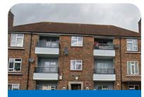
Concrete balconies with no thermal breaks allowing the internal walls to suffer low thermal performance
